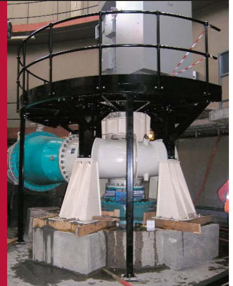
Figure 4: Bedford Pumps DV.90.23.10 Volute pump
