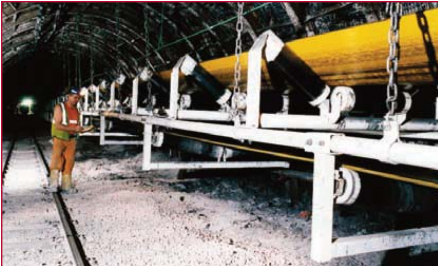
Figure 2: Underground engineers keep a keen eye on vibration levels
